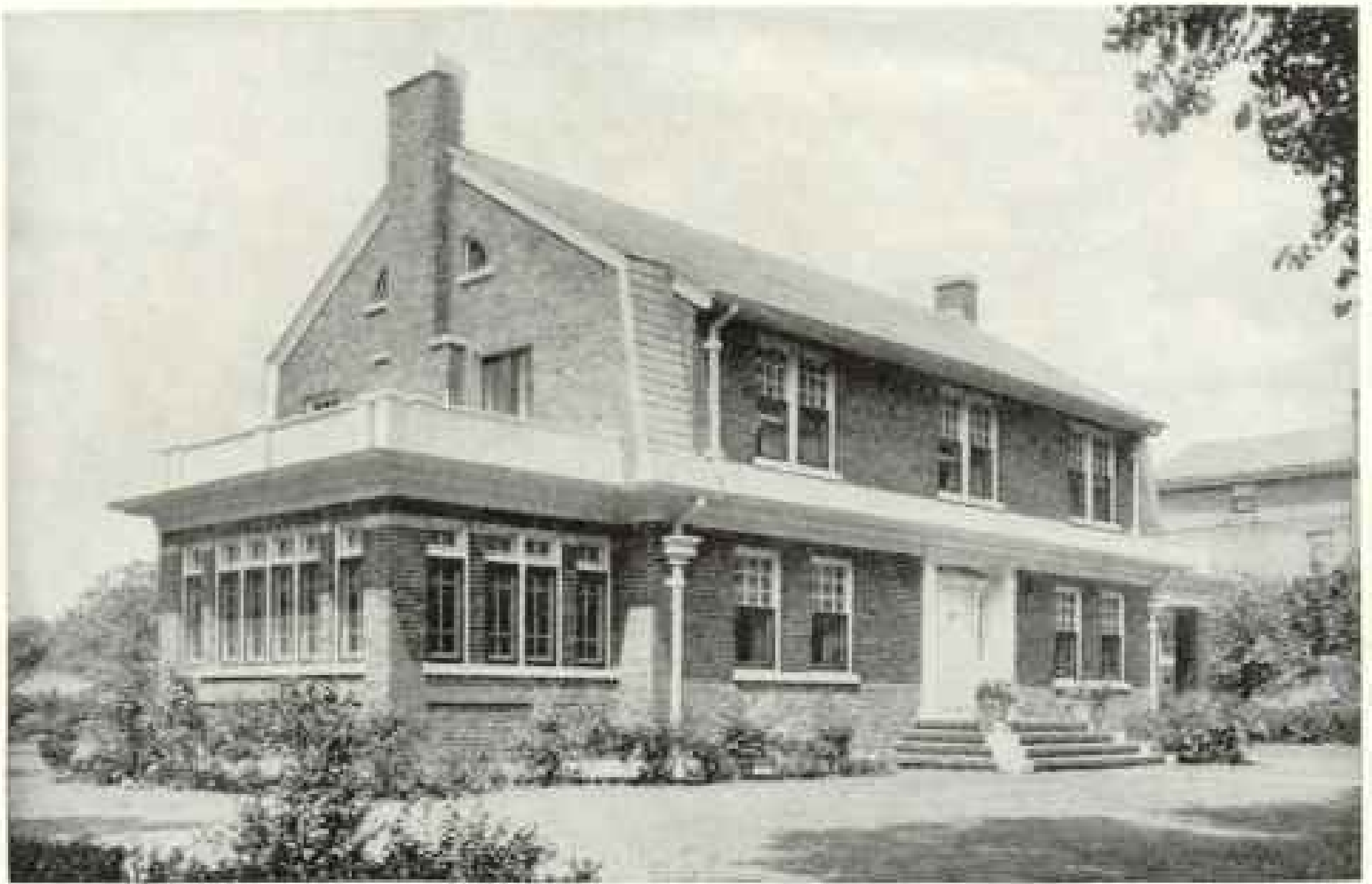
House at Chicago. Paul F. Olsen, Architect
