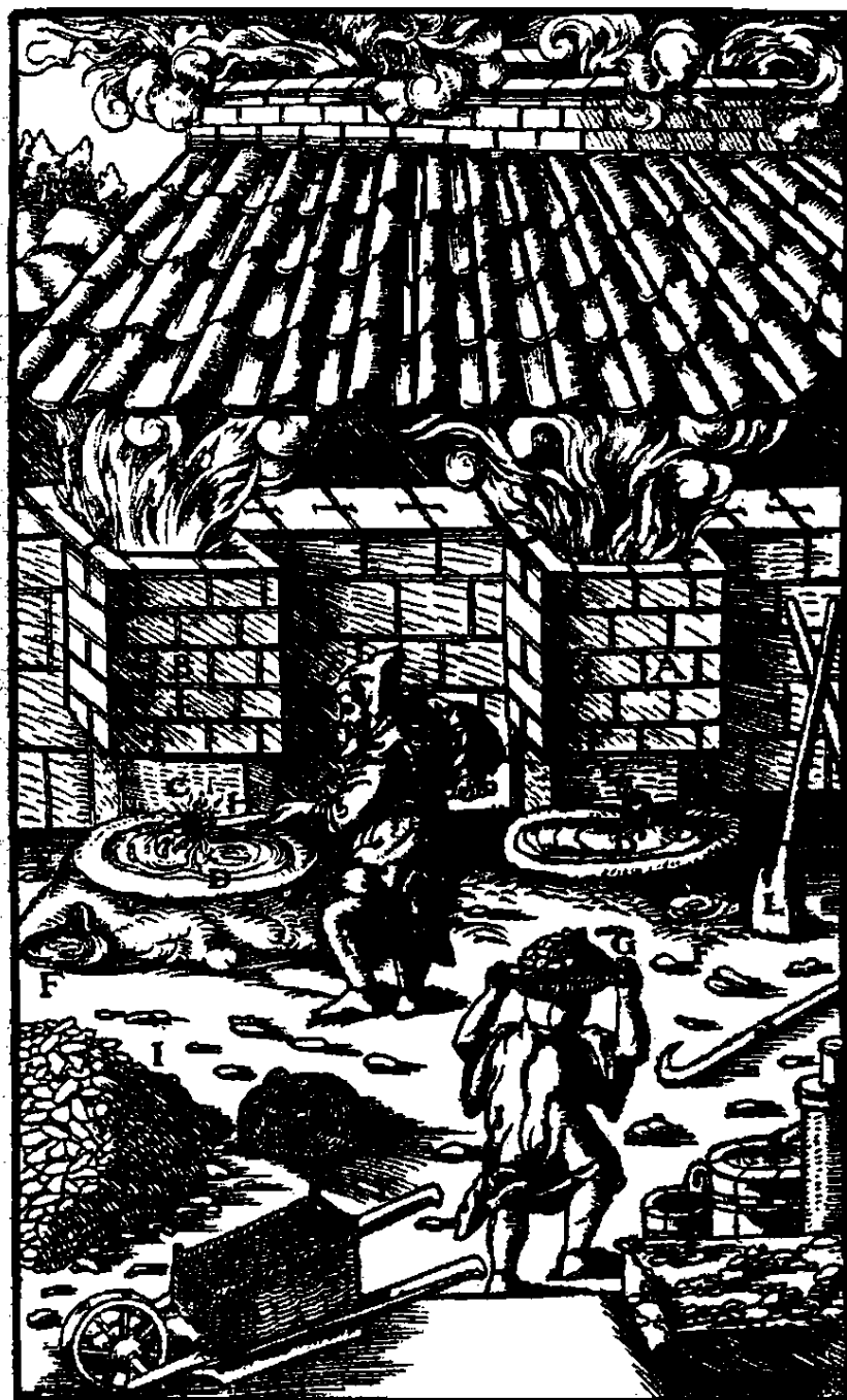
A, B—TWO FURNACES. C—TAP-HOLES OF FURNACES. D—FOREHEARTS. E—THIRD TAP-HOLES. F—DIPPING-POTS. G—AT THE ONE FURNACE STANDS THE SMELTER CARRYING A WICKER BASKET FULL OF CHARCOAL. AT THE OTHER FURNACE STANDS A SMELTER WHO WITH THE THIRD HOOKED BAR BREAKS AWAY THE MATERIAL WHICH HAS FROZEN THE TAP-HOLE OF THE FURNACE. H—HOOKED BAR. I—HEAP OF CHARCOAL. K—BARROW ON WHICH IS A BOX MADE OF WICKER WORK IN WHICH THE COALS ARE MEASURED. L—IRON SPADE.
